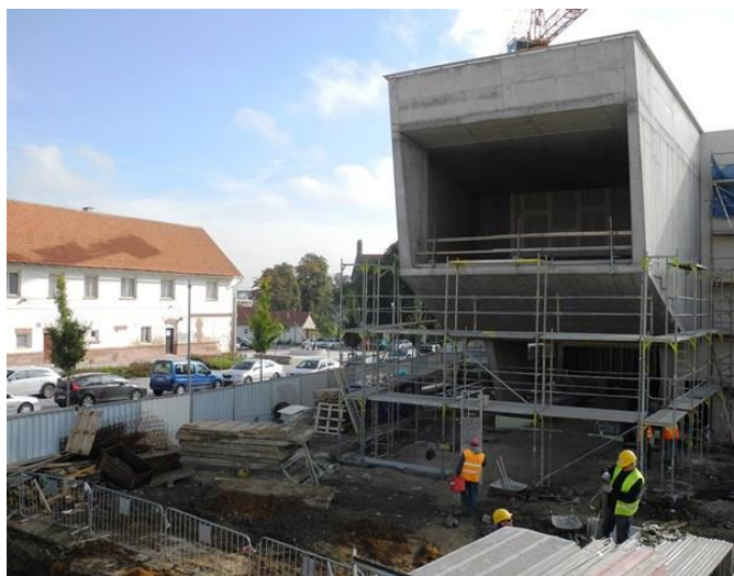
2013 – Construction of the HiLASE Centre building
