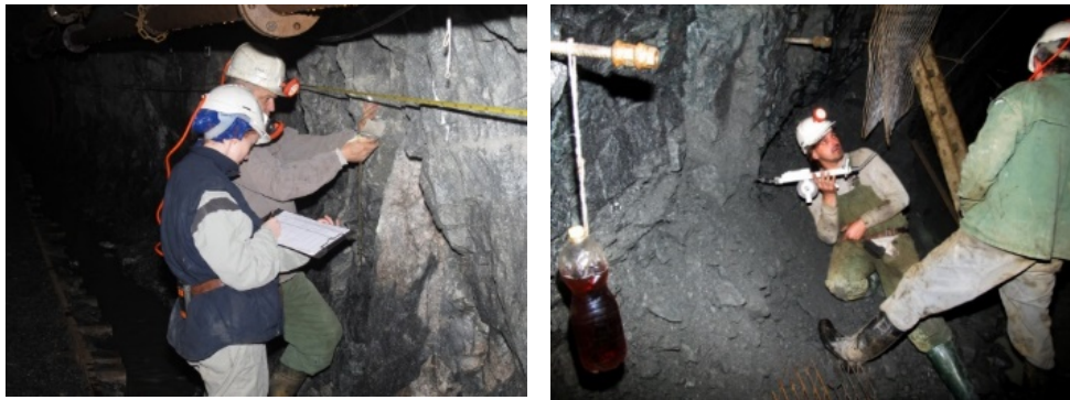
Fig. 7 Structural-geological mapping of mining facility walls for the purposes of determination of the rock mass quality (left) and convergence measurement (right)
